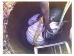
Prior to the application of the Ultra Bond III, Kelley and his crew used a 400,000 BTU ducted heater to pump heat into the manhole. This dry, hot air took the moisture out of the manhole structure and raised the temperature to about 90°F inside the manhole," says Kelley.
