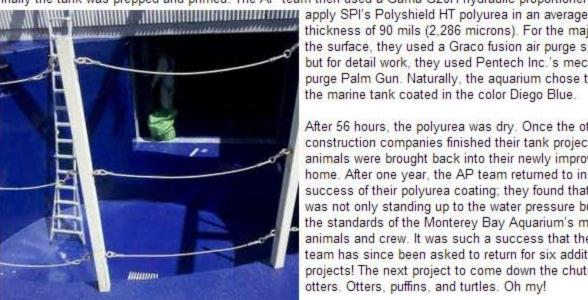
thickness of 90 mils (2,286 microns). For the majority of the surface, they used a Graco fusion air purge spray gun, but for detail work, they used Pentech Inc.'s mechanical purge Palm Gun. Naturally, the aquarium chose to have the marine tank coated in the color Diego Blue.
