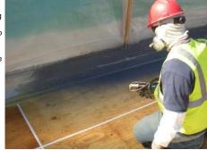
Two layers of 3/4" fire-rated plywood were then glued and screwed leaving a 1" gap around the perimeter and 6' around the drains for sloping. Then, "we sprayed the 8 lb. density Enveloseal SPF using a Gusmer 18/18 and ground the rough shape with a Calman Industries foam plane, finishing with a Clarke floor sander, Meyers says. "For the parapet to floor transition, we used 1" backer rod with Jaeger Tape to allow for expansion and contraction.
