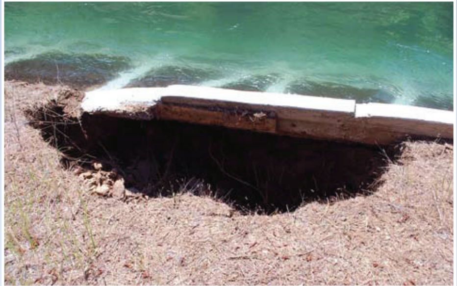
Void in the canal bank and intact lining.
