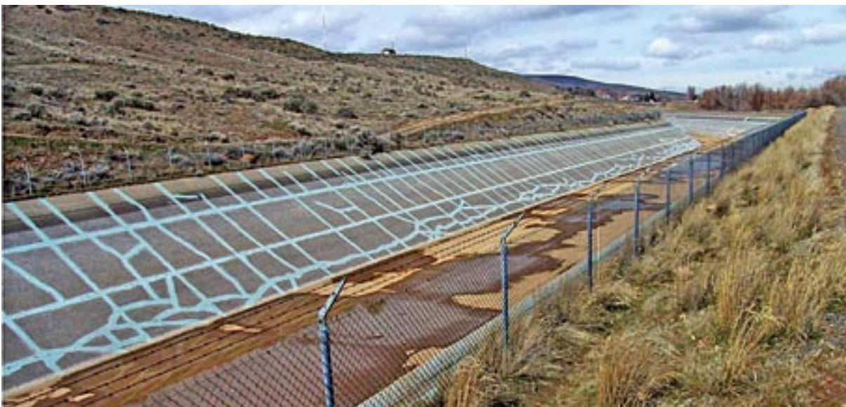
Polyurea coatings used at a water irrigation canal repair project.
