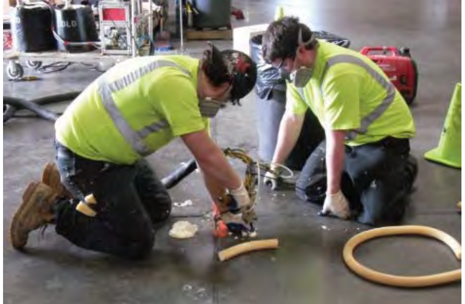
• • Synergy Series foam being used during a joint filling application
